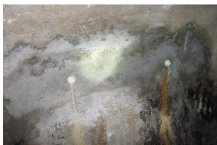
Previous leak repair
